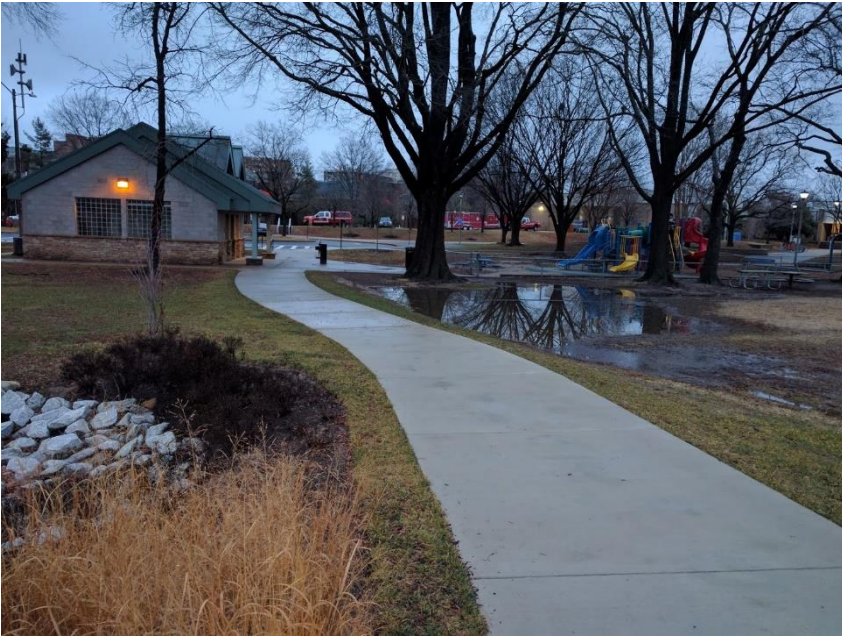
Figure 1 rain garden located on the left side of photo. Severe and deep puddling on the right side.
